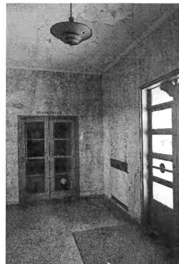
Figure 7: Doors to office wing from at left and entrance doors from Park Road at right.
