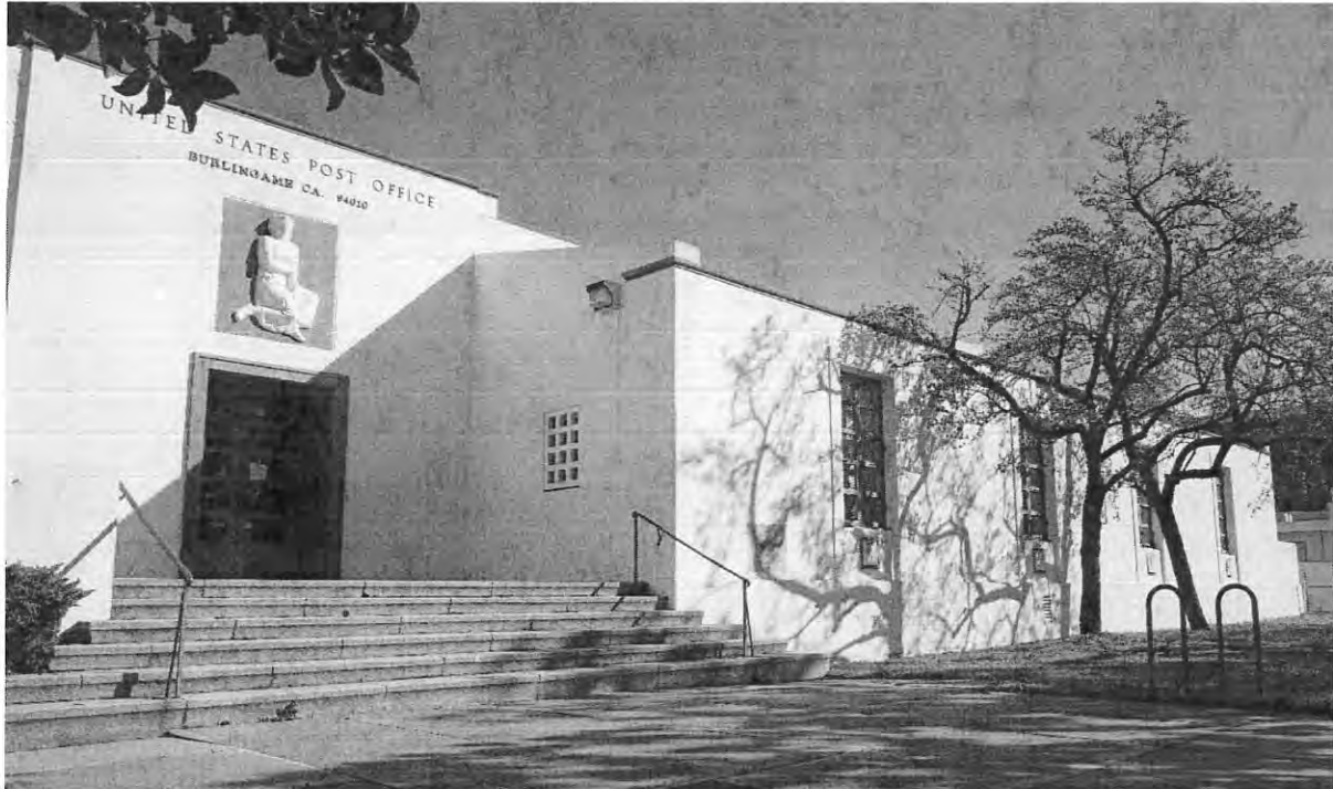
Figure 2: Park Road (southwest) façade, looking northeast.
